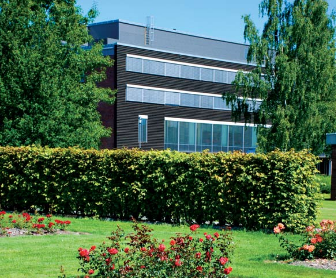
Norwegian University of Life Sciences with Jets™ sanitary system. Photo: Knut Werner Lindeberg Alsén
